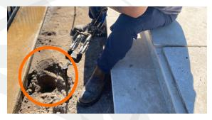
As technician injects I&I Guard - SSF into void behind seawall, signs of soil erosion were evident.
