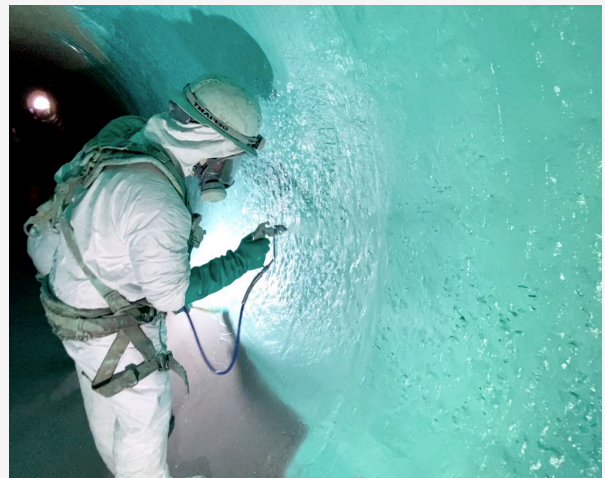
Structure Guard is spray applied using a dual component spray application system to achieve a consistent thickness of 250 mils throughout the pipe.
