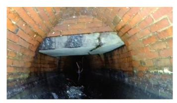
Before: The effects of age and corrosion caused the brick sewer to leak in critical sections of this tunnel, including three headwall obstructions.
