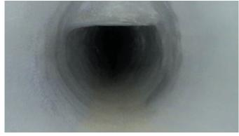
After: 1.75" of QLS GeoKrete was spray-applied to the non-round areas of the tunnel and delivered the required structural and corrosion protection.
