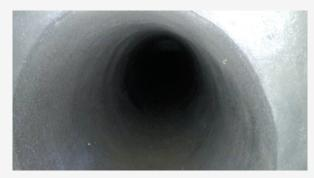
GeoKrete is precision applied in uniform thickness — resulting in a smooth, fully structural finish.
