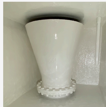
AFTER: Application of Structure Guard - Water at 80mils thickness.
