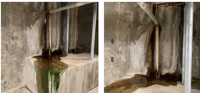
BEFORE: Water had begun leaking through multiple seams and puddling on heavily used walkways, creating a safety issue. Additionally, they identified a heavily corroded overflow weir used to ensure a uniform flow rate and avoid short-circuiting.
