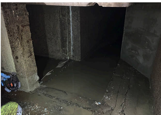
BEFORE: Wastewater Treatment Plant (WWTP) flume entry had begun to leak around the seams.
