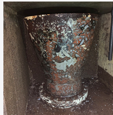
BEFORE: A weir was so corroded it was no longer functioning.
