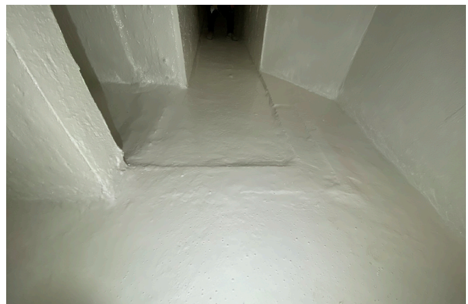
AFTER: WWTP After patching and sealing leaks with Hyperform®, the flume entry way fully rehabilitated with Structure Guard - Water.
