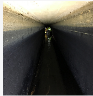
BEFORE: 100LF section of a 4' x 4' boxed-shaped potable water flume was leaking and creating safety issues along the walkway.
