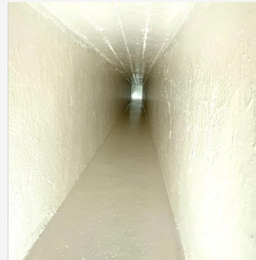
AFTER: After the voids and cracks were sealed with Hyperform®, the flume was coated with 80 mils of Structure Guard - Water for long term protection.
