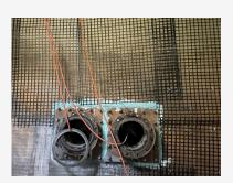
Carbon fiber reinforcement mesh was anchored within the GeoKrete® for added strength and stability.
