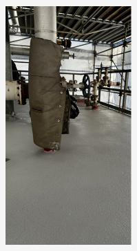
Oil stains and cracks in the original concrete on top of the structures coated with first application of Quadex E240 Epoxy and broadcast with quartz.
