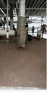
Final patched, repaired top exterior of basin, coated with final application of Quadex E100 Epoxy topcoat and Quadex E240 Epoxy and broadcast quartz applications.
